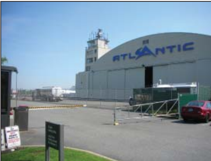
DW Smith Associates provided construction management for hangar renovations at Teterboro Airport.
